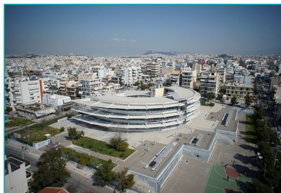
Building retrofit in Agios Dimitrios. © Municipality of Agios Dimitrios
